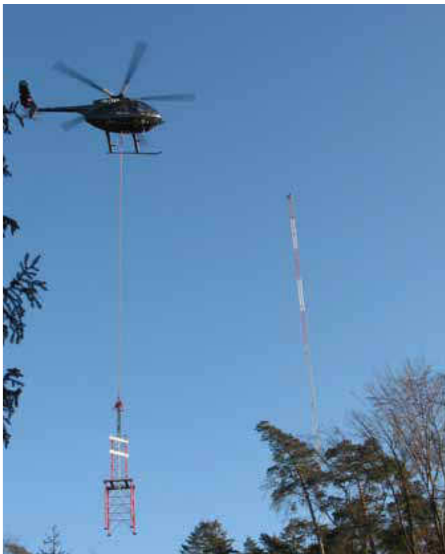
Figure 3: Construction of the 200 m wind met mast
