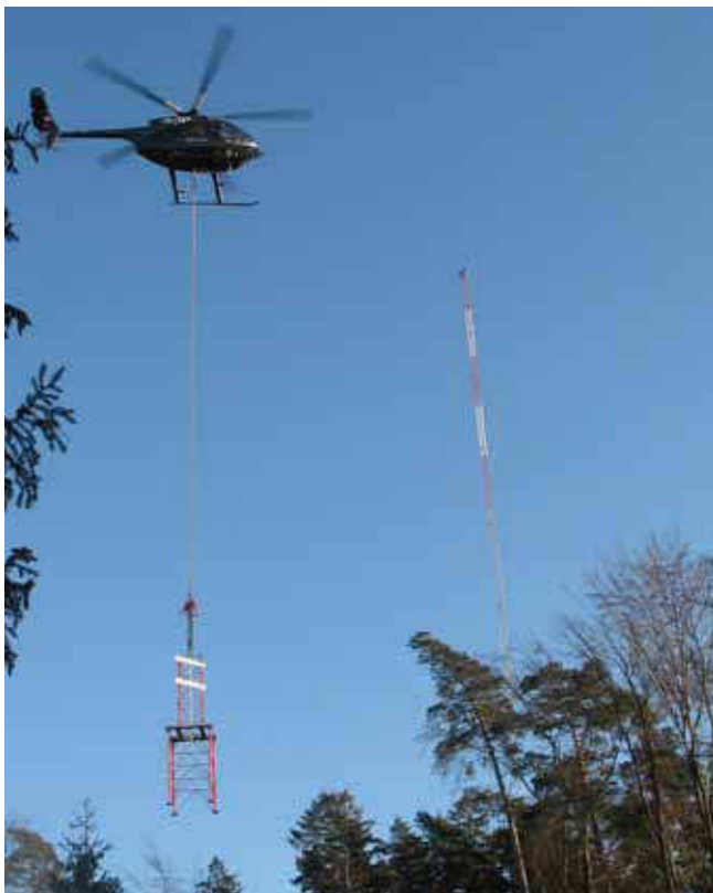
Figure 3: Construction of the 200 m wind met mast
